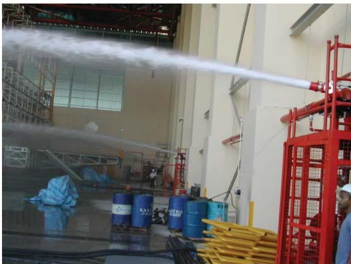
**Figure 12:** *Supplemental Protection for a Group I Aircraft Hangar.*
