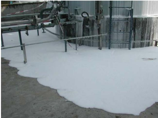
**Figure 7:** *Foam Blanket Spreading in a Diked Area.*
