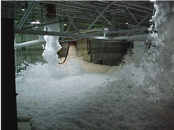
**Figure 8:** *High-Expansion Foam System Discharge. Photo Credit: Kidde Fire Fighting - National Foam*
