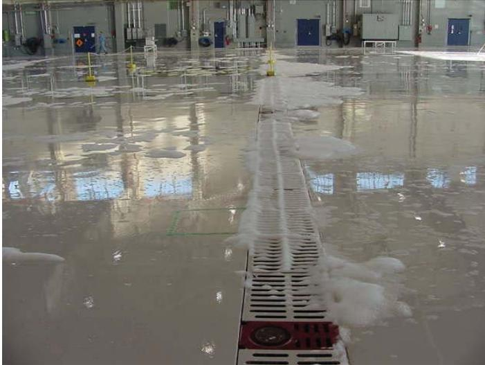
**Figure 11:** *Trench Drains in an Aircraft Hangar.*
