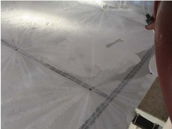
**Figure 10:** *Discharge of Low-Level Underwing Foam System.*
