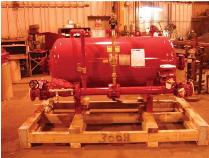
**Figure 1:** *Pre-Piped Foam System with Bladder Tank and Deluge Valve.*
