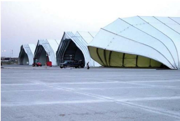
**Figure 13:** Example of a Class IV Hangar. Photo Credit: Public Domain --from Google
